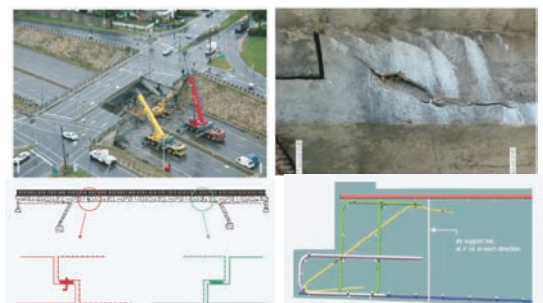
突然の橋梁崩壊事故：部材端部の劣化と不適切な施工と配筋 Commission of Inquiry into the Collapse of a Portion of the de la Concorde Overpass, Government du Quebec http://www.cevc.gouv.qc.ca/UserFiles/File/Rapport/report_eng.pdf
